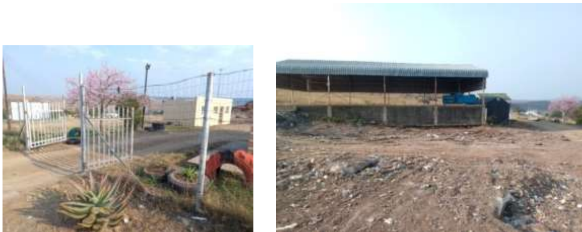
Figure9: Tsomo Transfer Station
